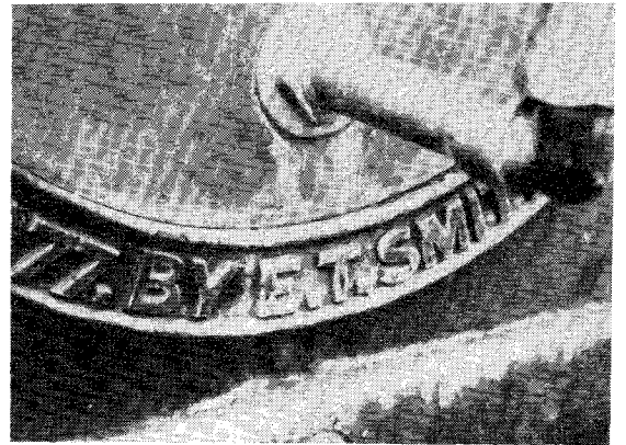
Figure 4 Section of a water fountain showing accelerated attack of the cast iron due to contact with a copper plate
