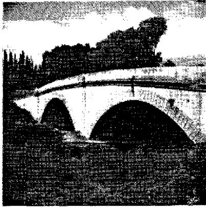
Figure 1 Waiakarua North Branch Bridge opened in 1874.
