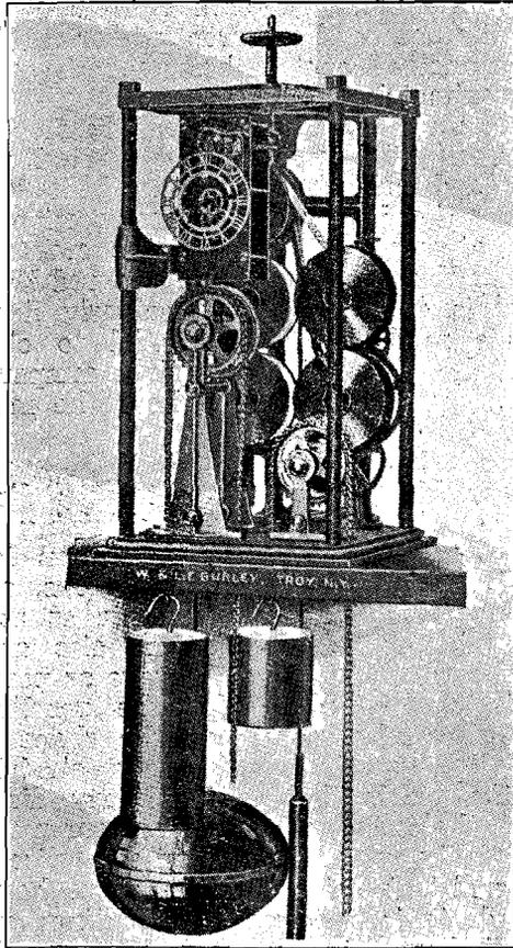
Fig. 4. Side View of Gurley Printing Water Stage Register, showing Paper Reels, Type Wheels, and Cushioned Hammers
